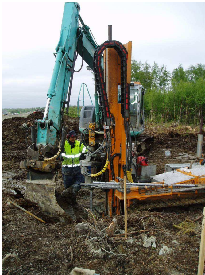
Figur 4-8. Pelarsondering.
